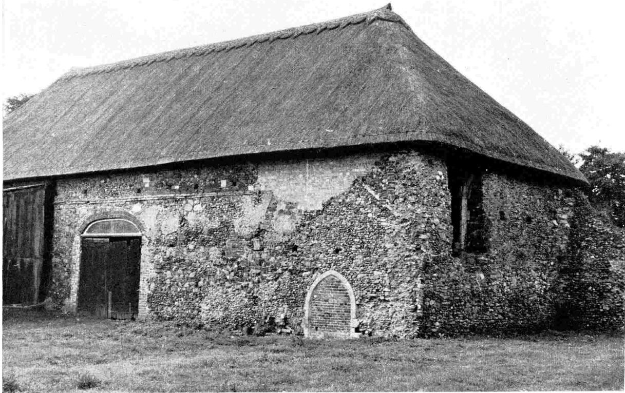
Campsea Ash Priory, barn (formerly part of west range) from north-east.
